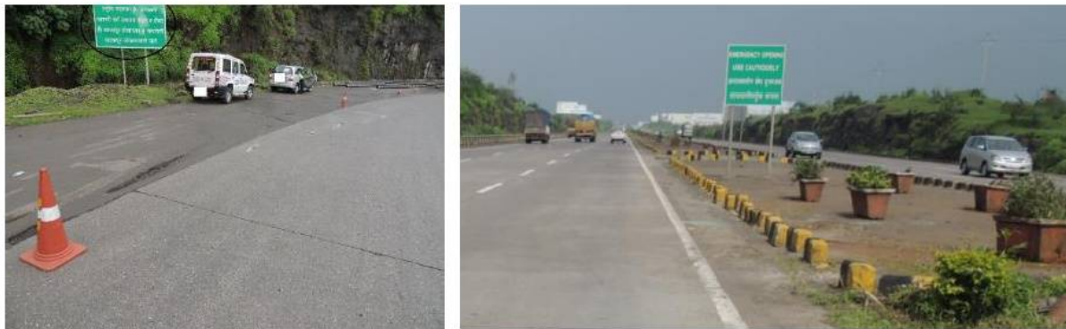
Figure 9 examples of poor/ineffective road signage on the expressway
