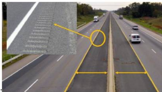
Figure 4: shoulders provided on both sides of the roadway (road side and median side) with continuous rumble strips, to prevent use of shoulders as regular travel lanesSS
