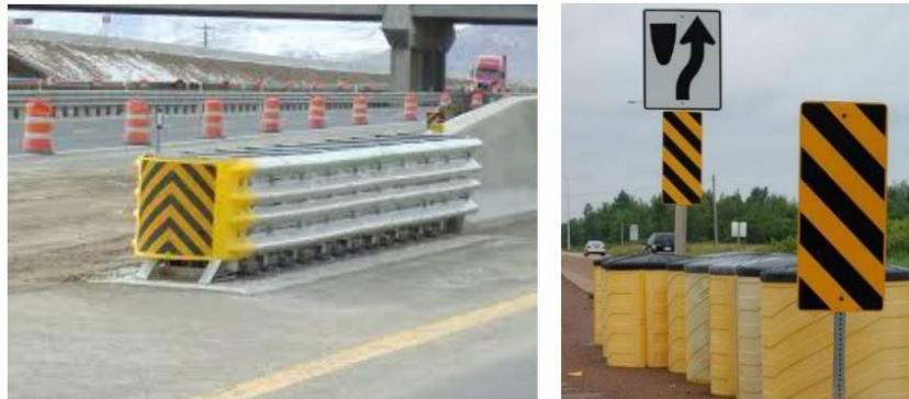
Figure 6: pictures of impact attenuators – metal (left) and sand/water- filled barrels (right).
